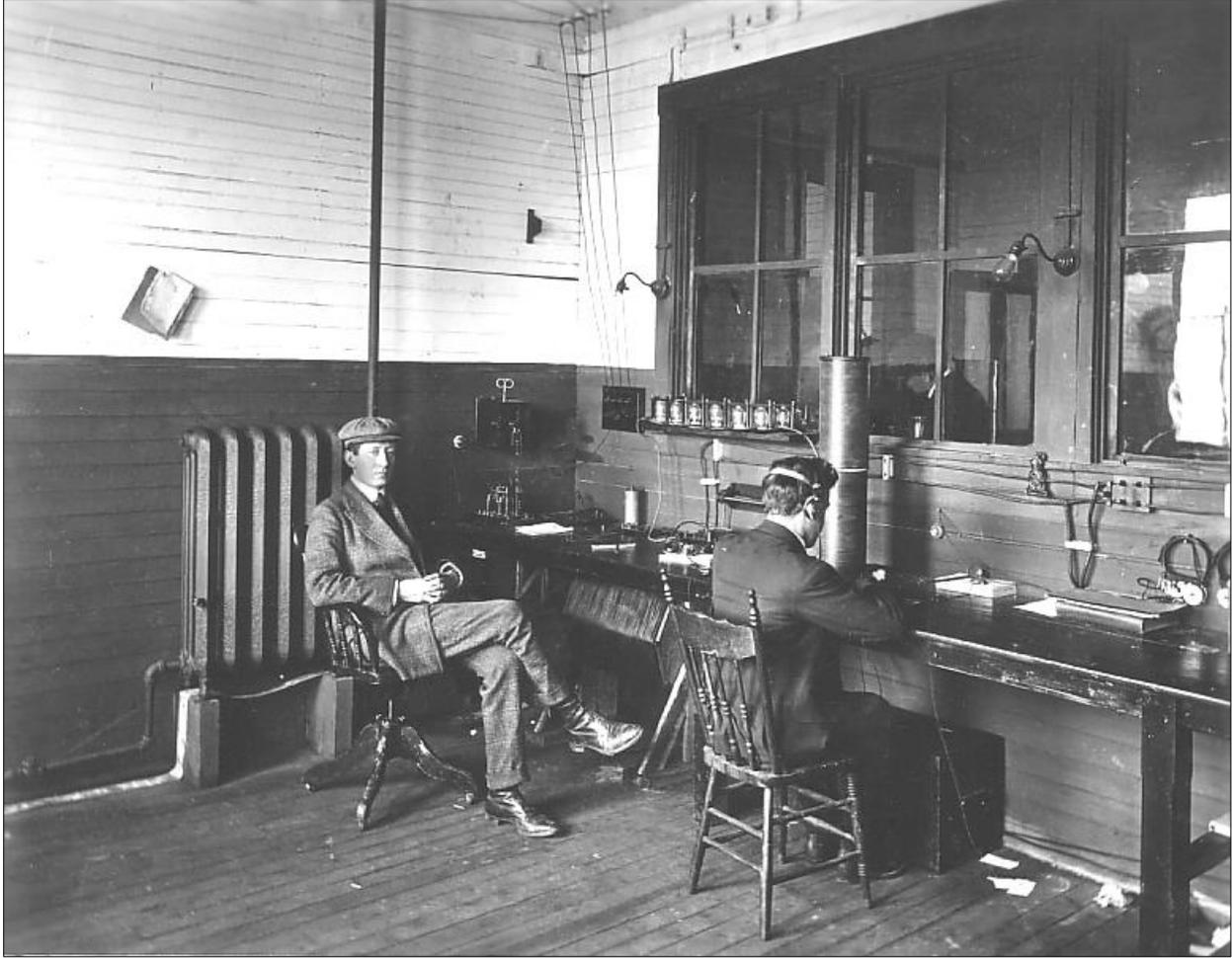
**Marconi used Fleming Valve as detectors in the Glace Bay station as early as 1907; a row of 7 spare Fleming valves can be seen lined up to the left of the wireless operator. Marconi is seated on the left**
