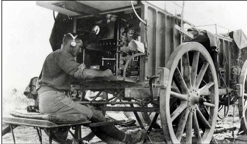
**One of the first tactical transmitter-receiver set made by Marconi UK, with its Royal Engineers Signal Service operator (1500W transmitter version)**
