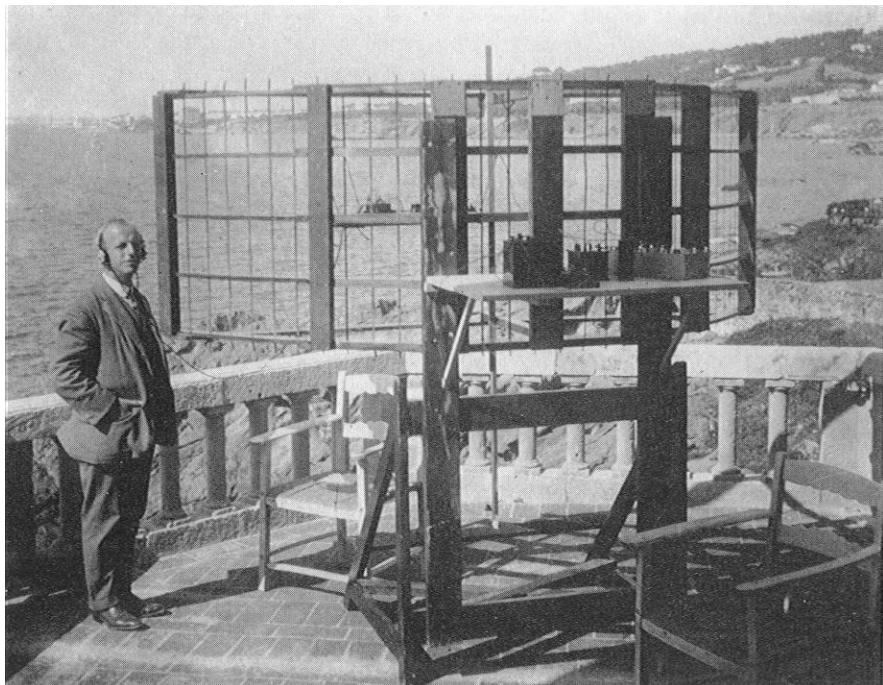
C.S. Franklin of the Marconi Co. with the first short wave directional aerial working at 2 meters in 1916.
